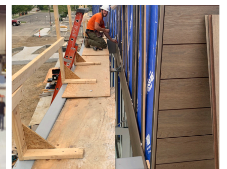
Happy installer on site.
